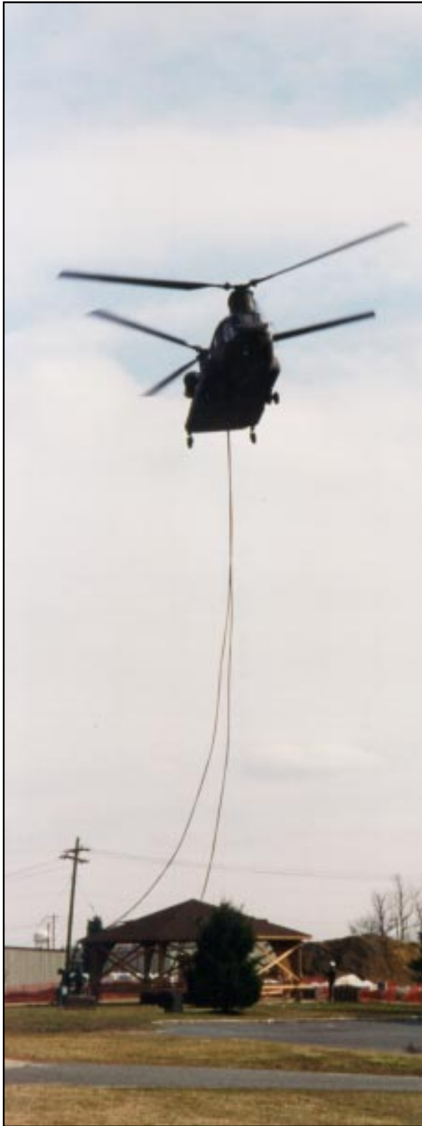
The “Nomads” of G Company, 104th Aviation, recently made short work of placing two 20,000-lb. gazebos near the Airman Leadership School at McGuire, Air Force Base in New Jersey. Moving the gazebos by air saved the Air Force the time and expense of tearing down and rebuilding both structures at the school. □
