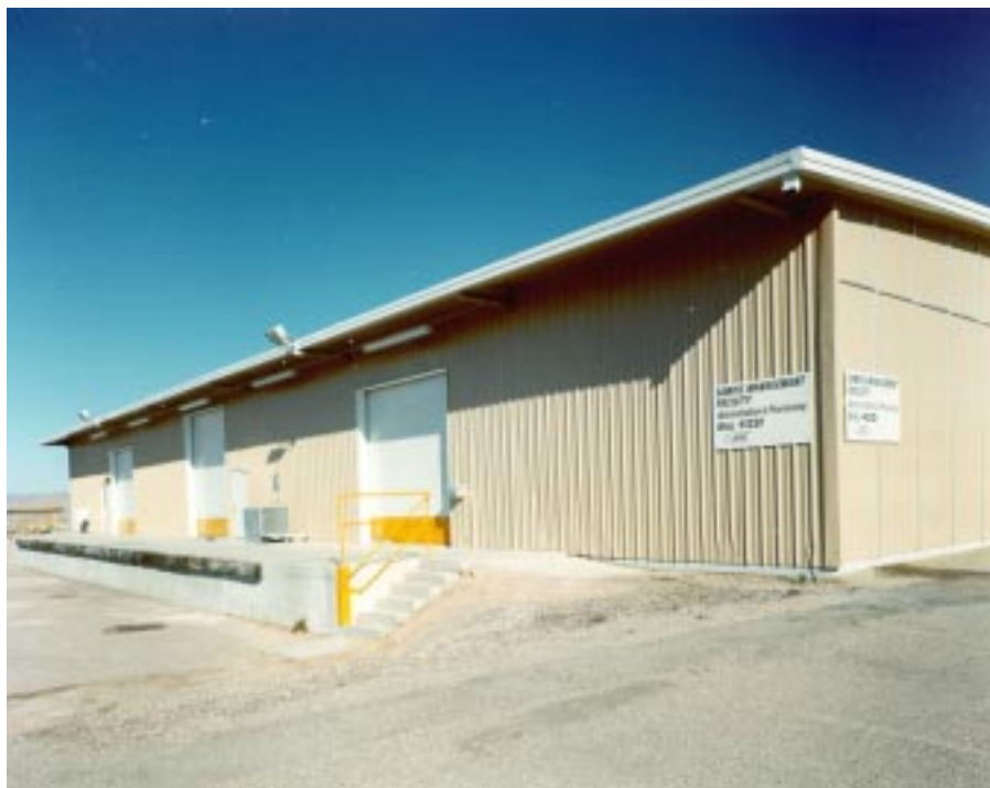
QA Sample Management Facility at Yucca Mountain
