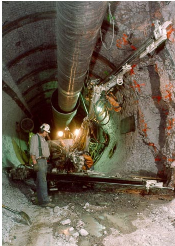
Drilling in Alcove 8
