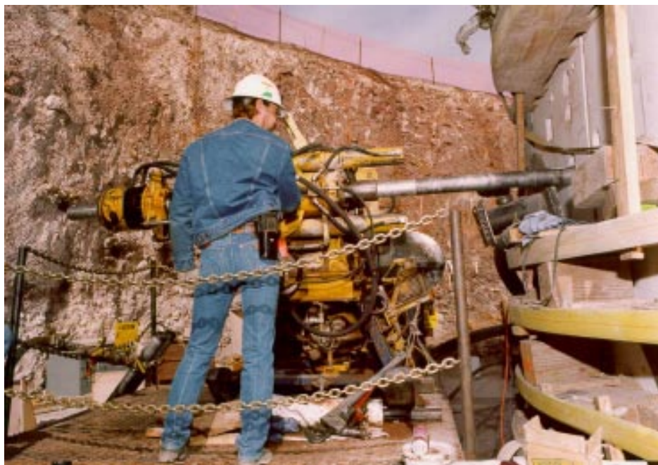
Large block heater test
