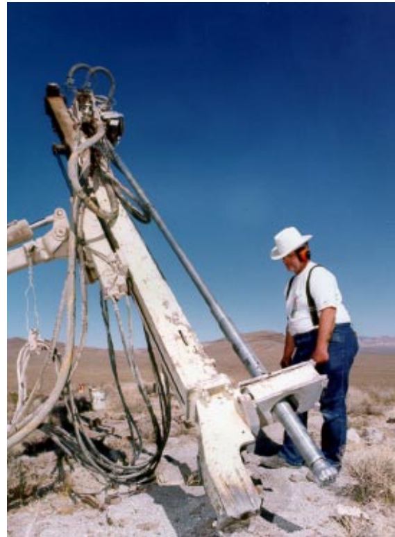
Constructing a monitoring station at Crater Flat
