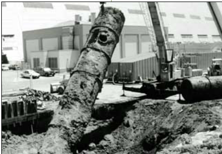
Leaking underground storage tanks are the most common source of groundwater contamination in the United States. New requirements in 1998 required that all petroleum underground storage tanks meet comprehensive corrosion, spill, and overflow protection upgrades.
