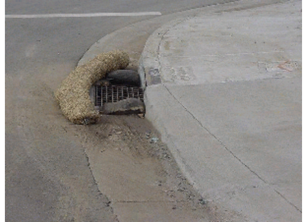
Control of sediment into storm drain
