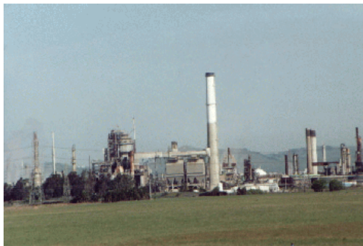
Refinery in Northern California, a major discharger
