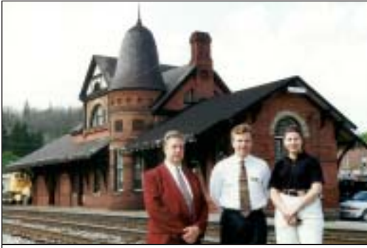
B&O Railroad Station Renovation and Rehabilitation in Oakland, Maryland
